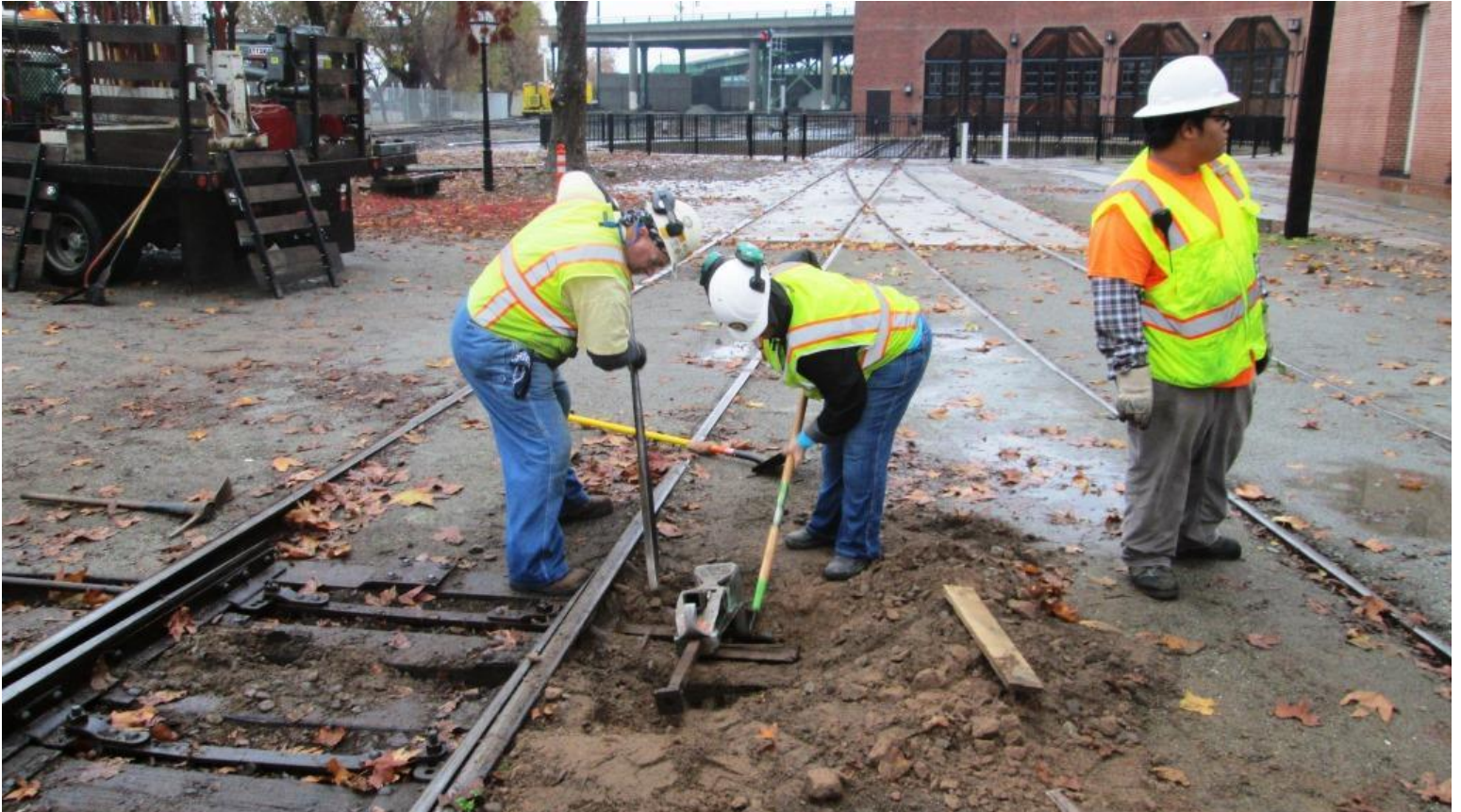
Once the tie is moved, Mike F. and Pam pack dirt under the tie to hold it in place
