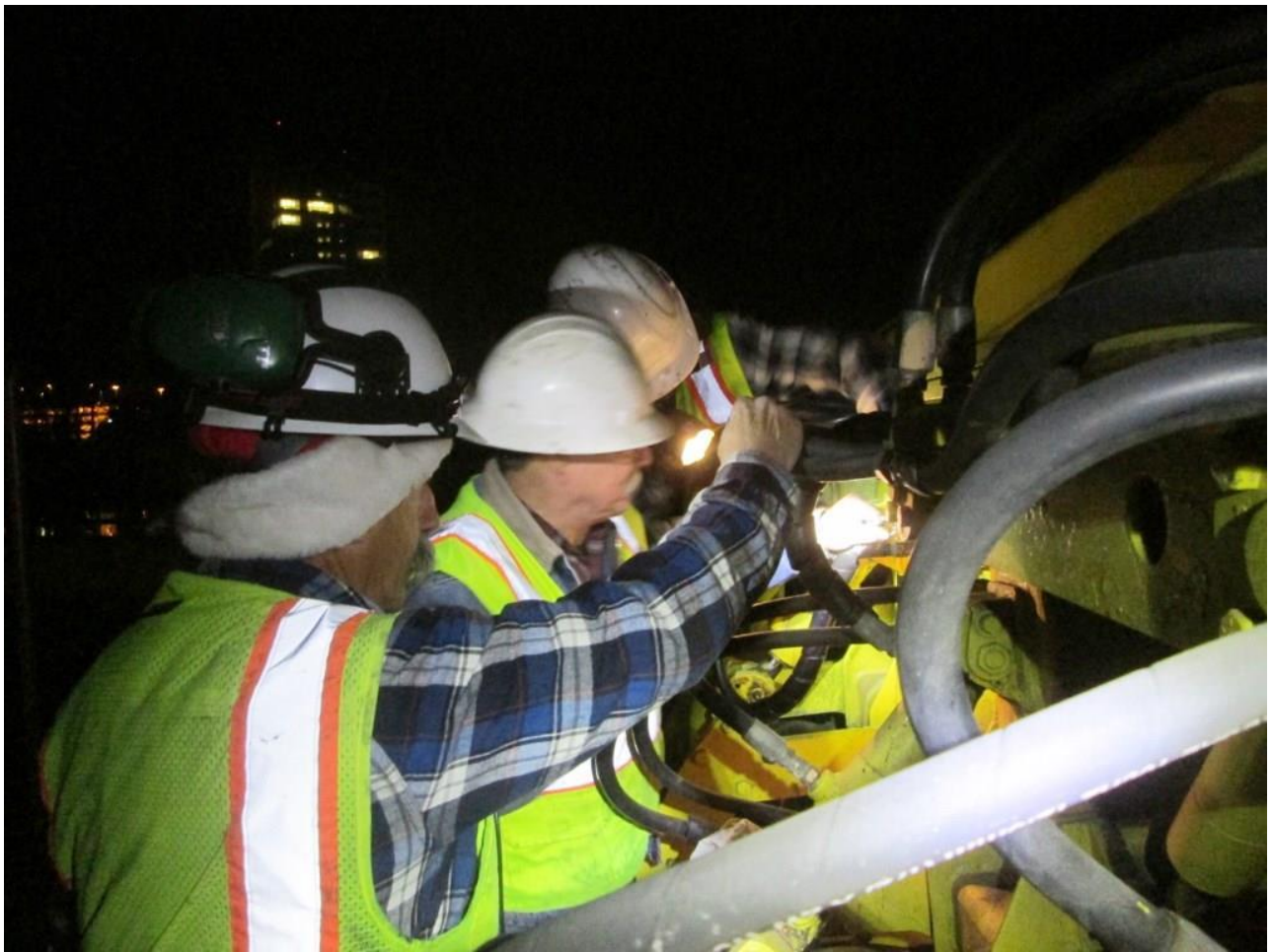
Joe, Mike H., and Matt remove hydraulic hoses from the offending vibrating motors
