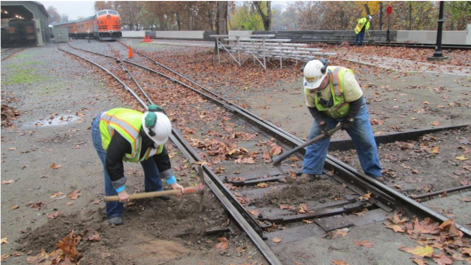
Pam and Mike F. loosen the soil-cement around the tie to be moved
