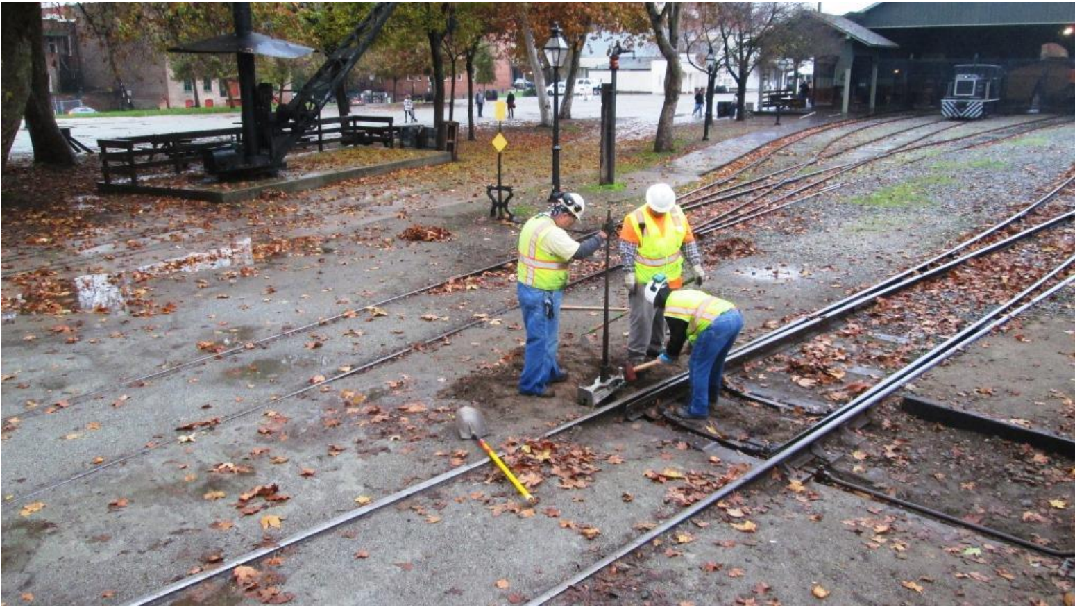
As Mike F. cranks on the jack, Pam strikes the bracket with the sledge hammer to help it slide
